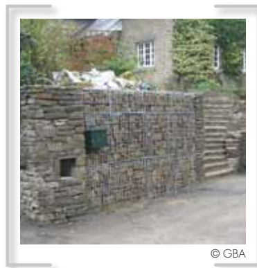
Dallage, couvre-mur, gabions
